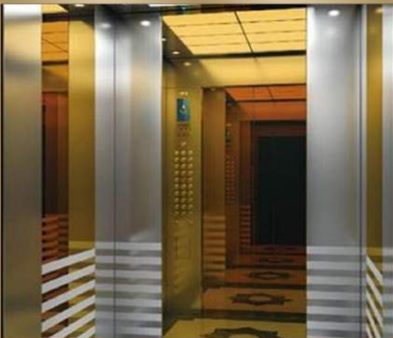
High Speed Golden Elevators
